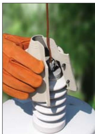
Rubber Glove Installation of R-21116
